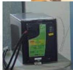
TLC battery 48 V-4 kWh
