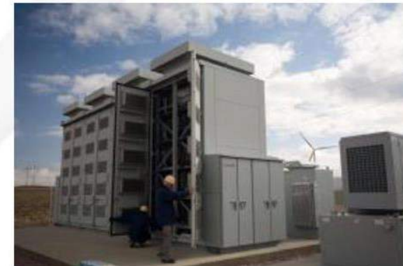
Grid-connected ESS Na/S 1 MW – 7,2 MWh
